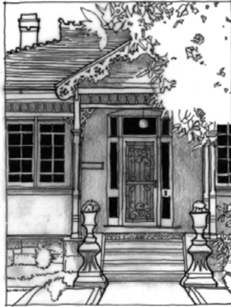
Part D - Figure 21: Intricate timber detailing to gable ends, verandah posts, brackets and frieze are contrasted with fine tuckpointed brickwork giving this Federation bungalow a high level of technical expertise of construction
